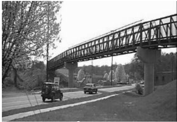
Lakewood Ave. Bridge, Durham County
