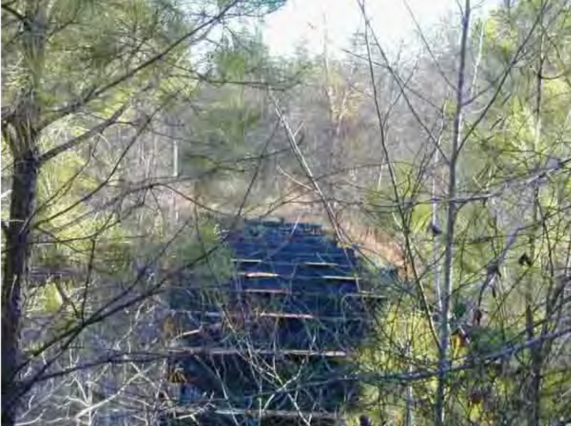
Bridge Structure Over Northeast Creek
