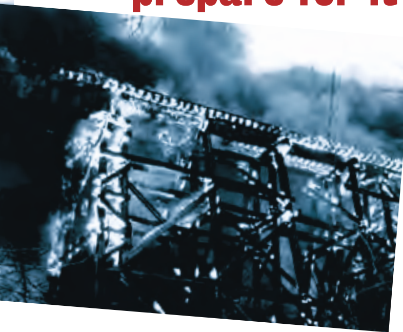
Pennsylvania's Kinzua Bridge (left) was devastated by a tornado. This fire in Maryland's Rock Creek Park was the result of arson. The trestle was repaired and is now on the Georgetown Branch Interim Trail.
